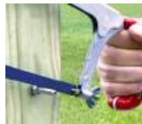
Step 2 Cut thread leaving 1/4"
