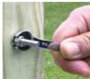
Step 1 Tighten nut to tension
