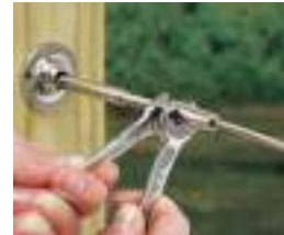
Tighten cone onto receiver.
