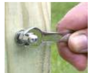
Step 3 Install acorn nut
