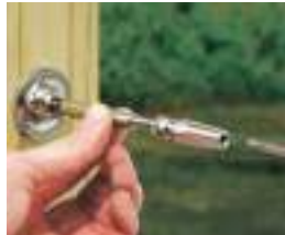
Fully seat wire rope.
